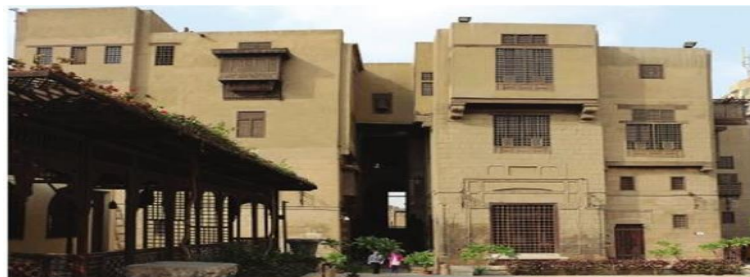
Figure 1 BAYT AL-KRITLIA BUILDING
